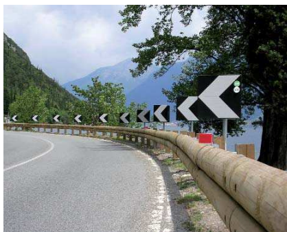
two half-round logs diameter 22 cm, length 4.00 m or 2.00 m reinforced steel U-profile at the rear.
